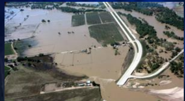
US Hwy 34 East of Greeley, 2013, CDOT
