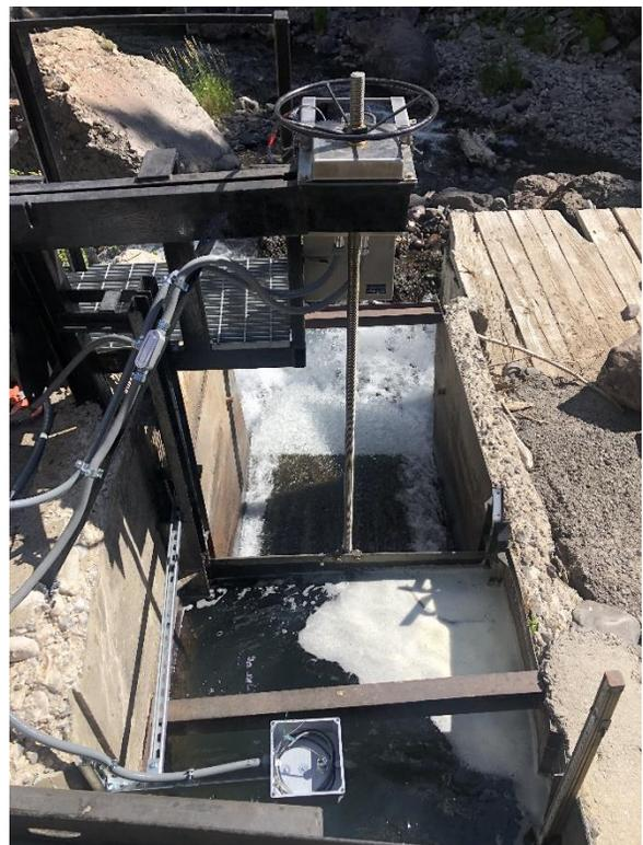
Waste gate with SCADA controlled motorized actuator. Photo: Allen Distel
