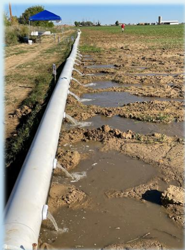
A series of 30' pipe sections laid out on the uphill side of the field
