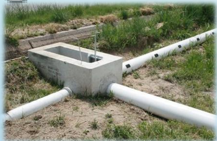
Water source channeled into a line of pipe
